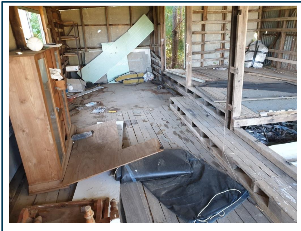
Photograph 4 - The interior of the shed.
