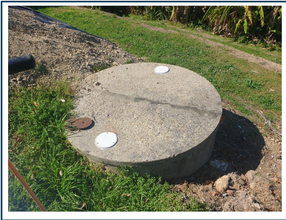
Photograph 1 – The existing concrete septic tank servicing the dwelling on proposed Lot 2.
